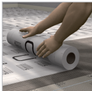
DRY-DF – sealing film for surfaces
