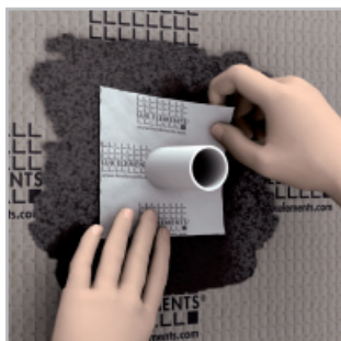
DRY-DBWM – sealing pipe duct
