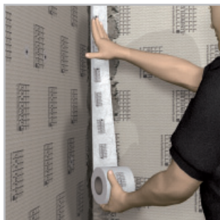
DRY-DB(V) – integrating sealing tape into wall/floor connections
